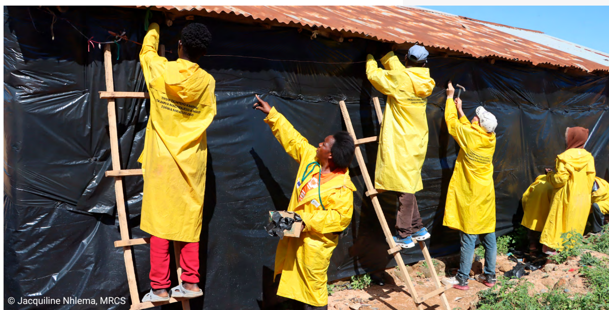
Members of Mzati GCT in Ndirande, Malawi cover a house with plastic to protect it from strong winds.
