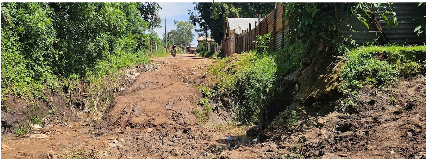
Photo 9.1: Erosion In A Thousand Street
