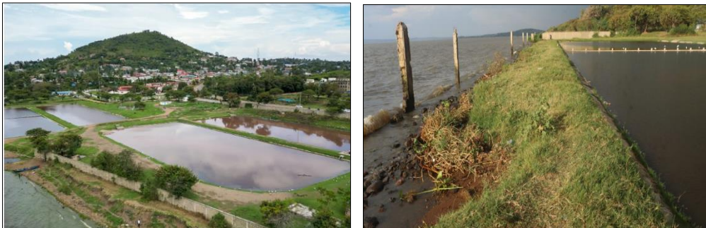
Figure 32: Homa Bay Sewerage Plant (Source: Global Partners for Development (left) and Kenya News(right))
