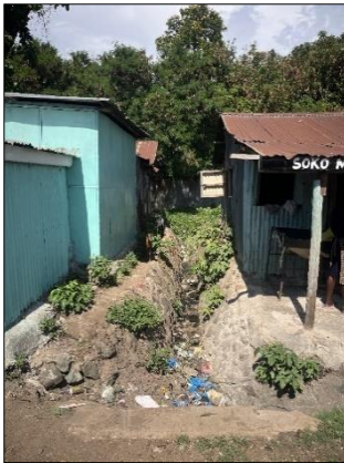
Figure 17: Drainage swale between buildings – Shauri Yako (SUEZ Consulting, 2025)
