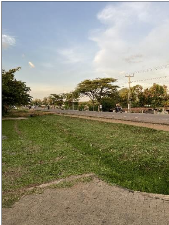
Figure 20: Drainage swale on the C19 roadside (SUEZ Consulting, 2025)
