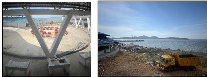
Figure 28: New fish market in construction (@SUEZ Consulting, 2025)
