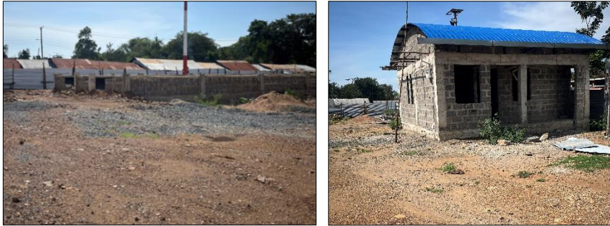
Figure 27: Rehabilitated market by KISIP in construction (@SUEZ Consulting, 2025)
