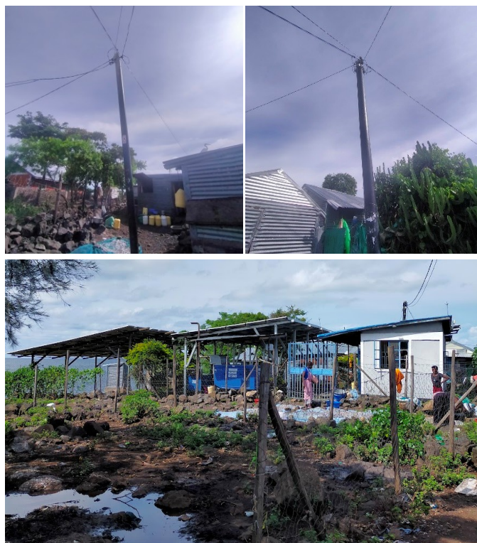
Photo 4 Solar Lighting Supply
