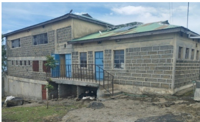
Photo 4.1: Ringiti dispensary. (Source: AMT field visit, 2025)
