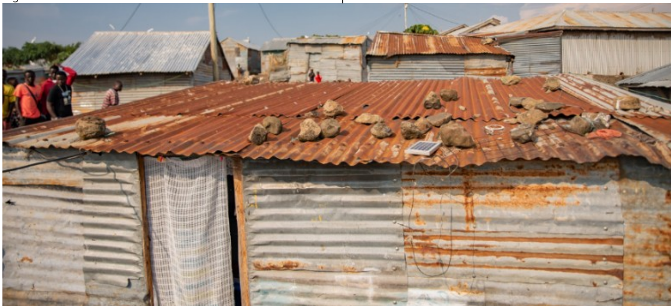
Photo 5.2: Informal Corrugated Iron Housing Secured with Stones on the Roof (Source: GCA field visit 2025)
